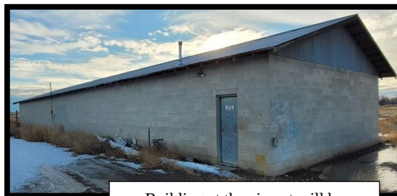
Building at the airport will be demolished for BLM SEAT Base.
