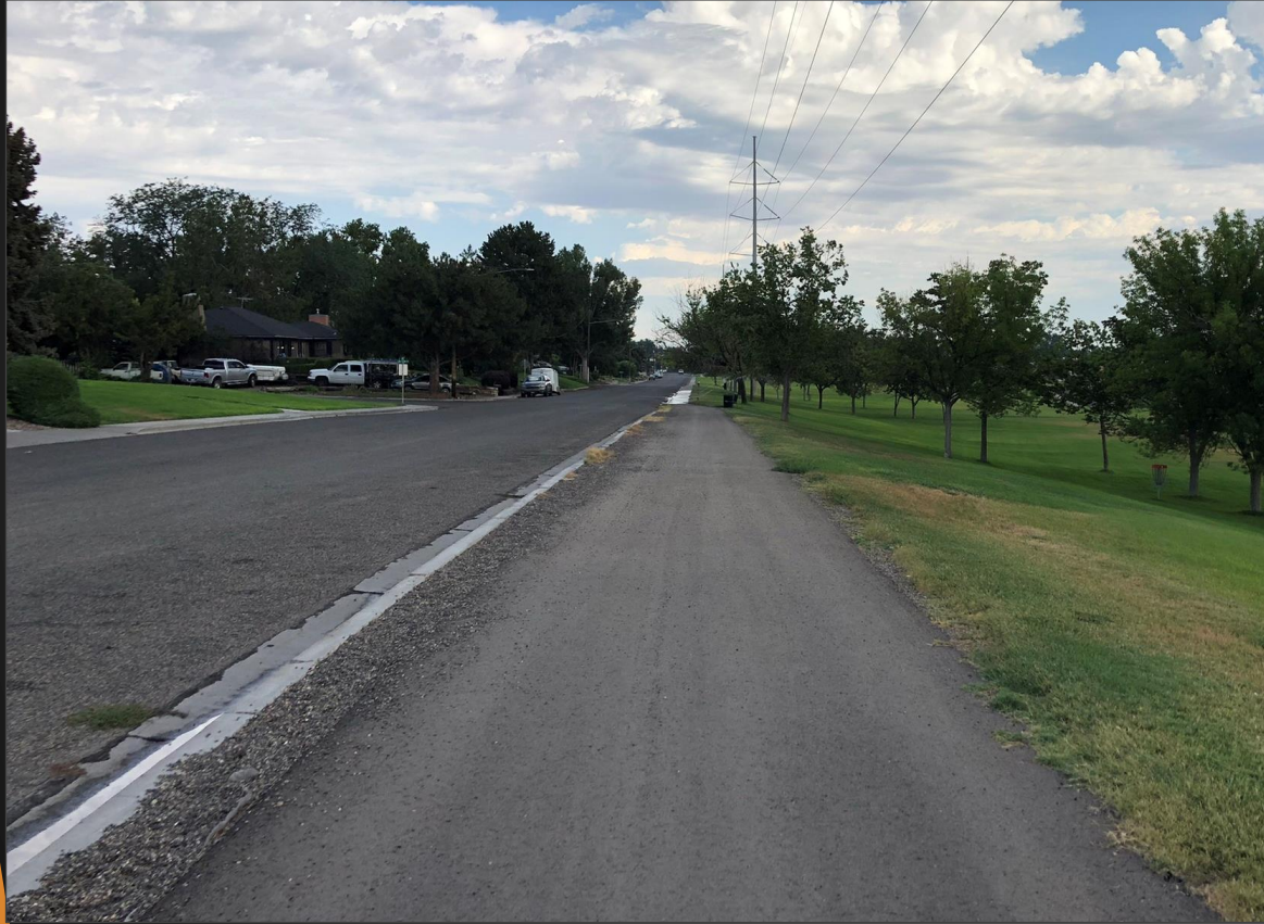
Adjacent to Street
