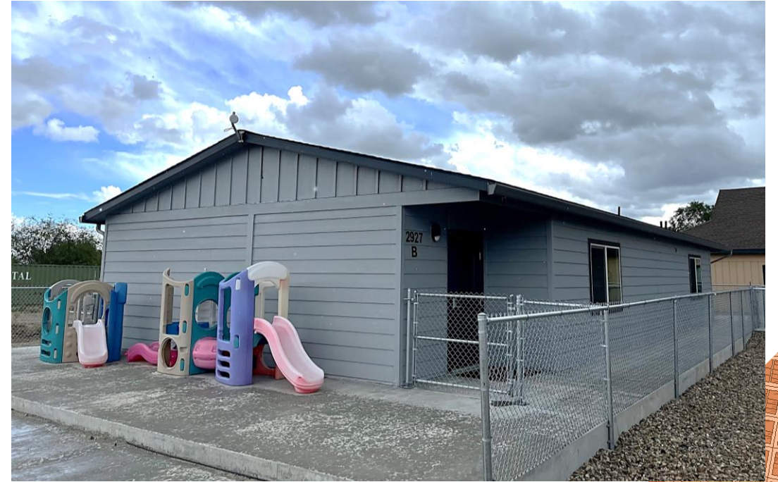
Completed: ESD Modular Classroom ESD Building, SW 6 th Avenue
