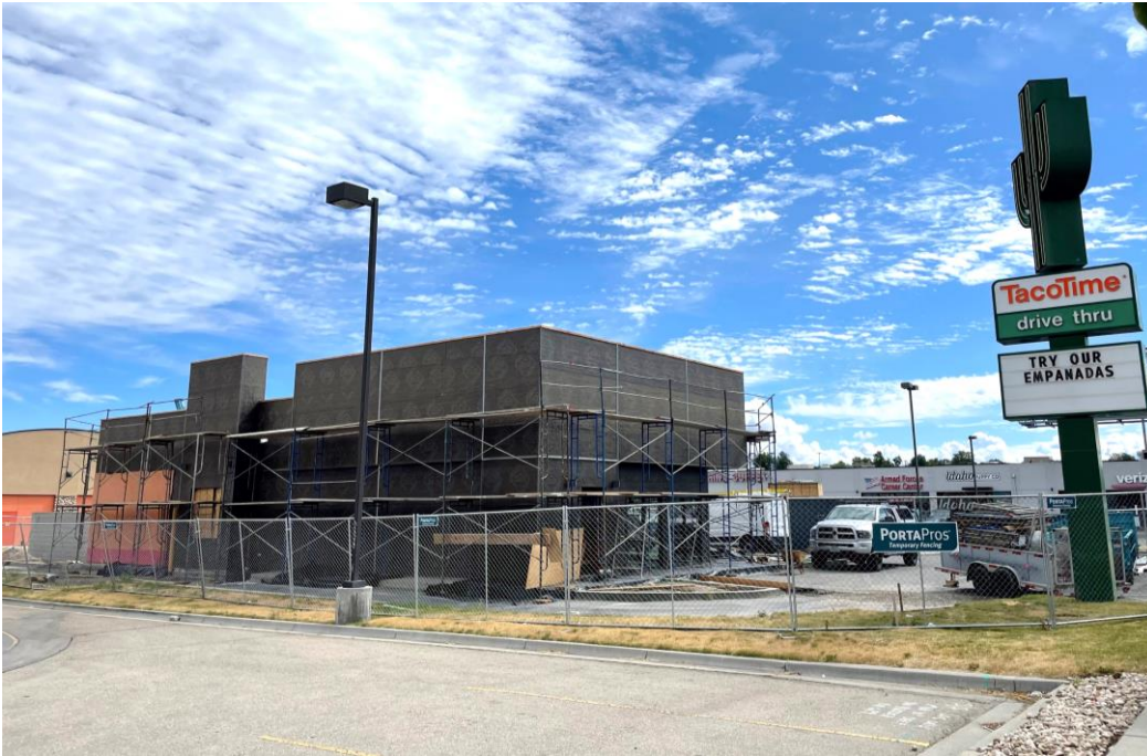
Under Construction: Chipotle Restaurant (Old Taco Time) West Idaho Avenue
