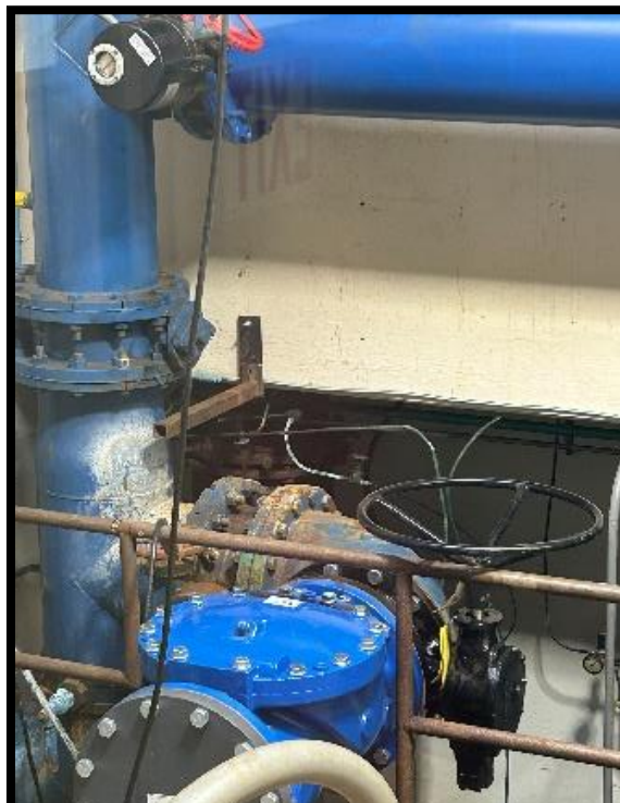
Installed new Butterfly Valve and Check Valve on clearwell pump 4 discharge line
