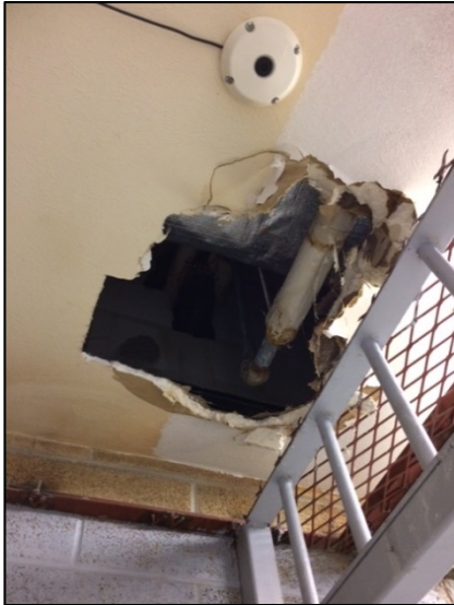
Water leak repaired in Ontario City Hall police holding cell.
