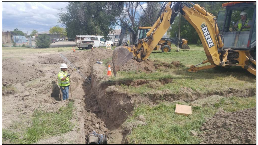
Field Services Crew digging trench for new water main water to new Well No. 17 at the Water Treatment Plant.
