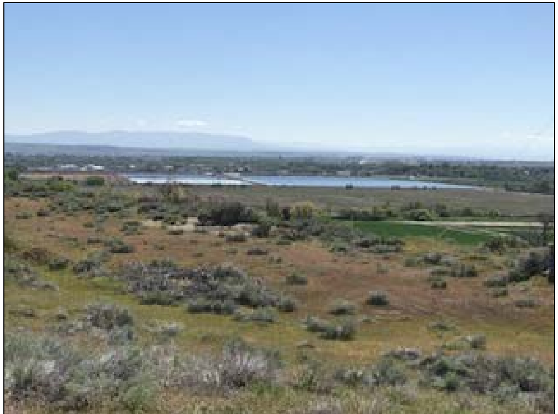
View of the Wastewater Treatment Plant lagoons from the Bench Reservoir.
