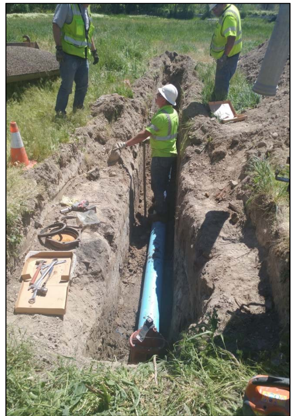
Field Services Crew installing new water valves to new Well No. 17 at the Water Treatment Plant.
