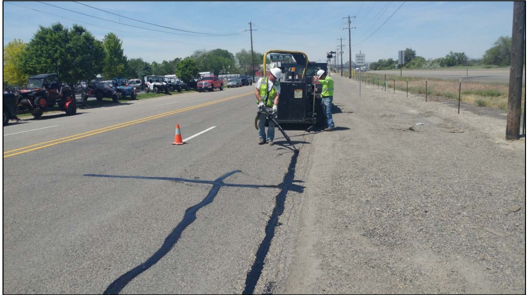
Field Services Crew crack sealing on North Oregon Street prior to chip seal project.
