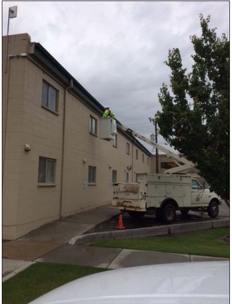
Parks and Cemetery/Facility Maintenance Crew mends rain gutters at the City Hall apartments.
