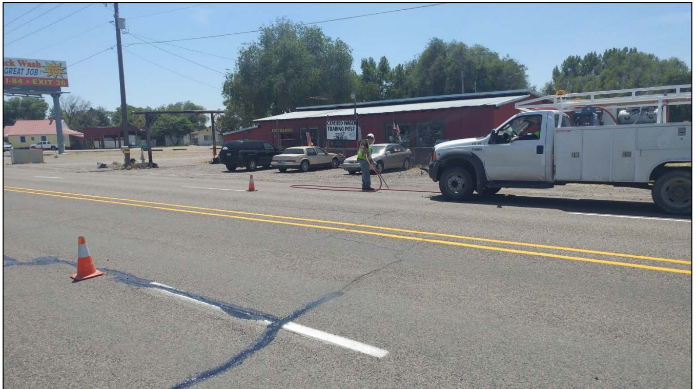
Field Services Crew blowing out the cracks in the asphalt before crack sealing crew follows.
