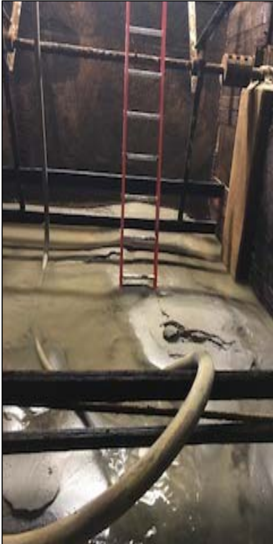
Water Treatment Plant Crew removing sand from Clarifier No. 2.
