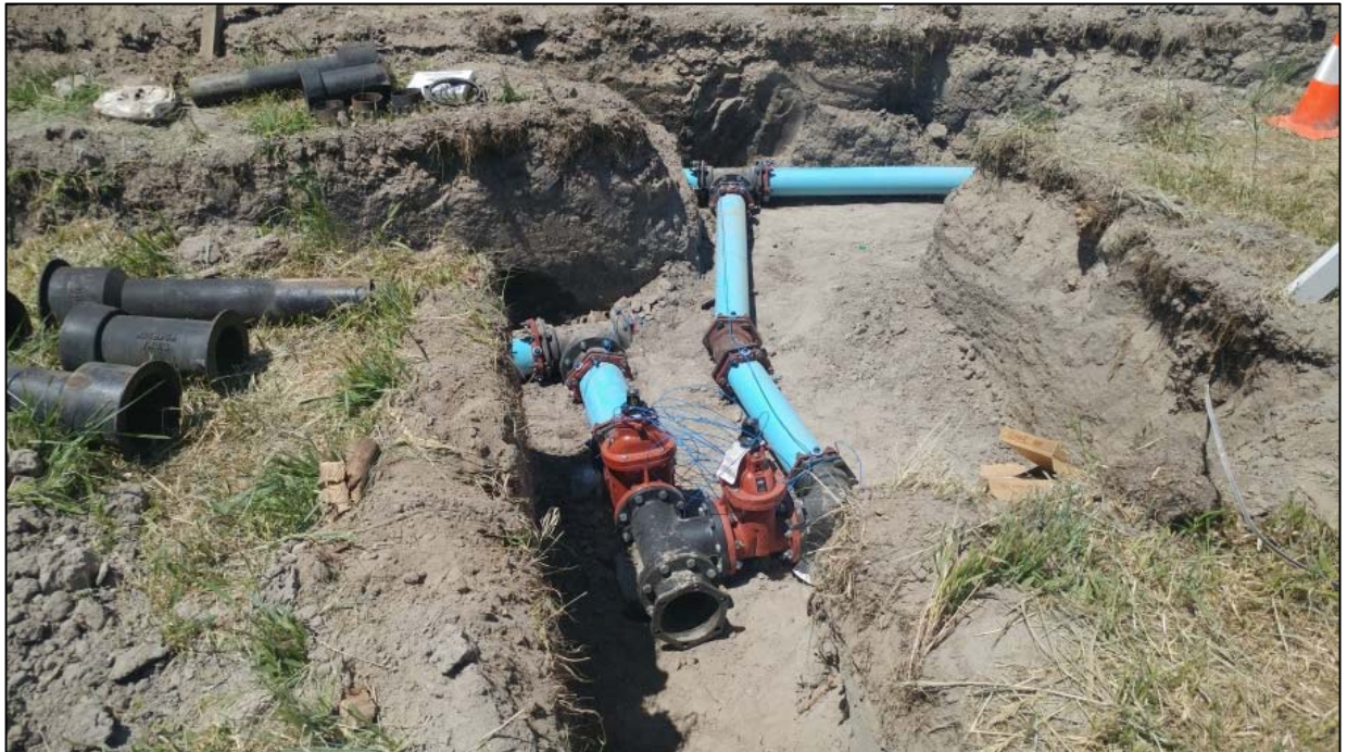
Above photos: Water Treatment Plant Well No. 17 new valves and tees installed by Field Services Crew.
