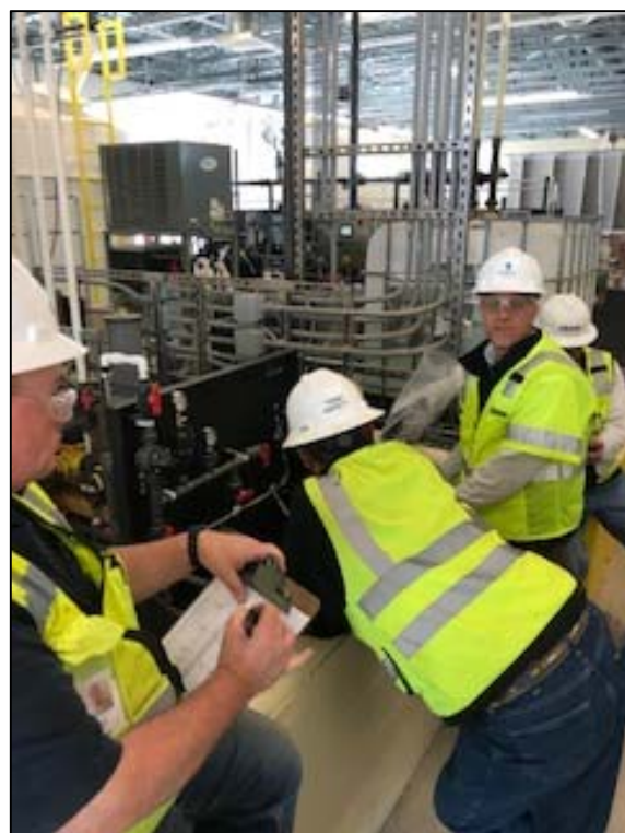
Crew running pump calibration curves for the new ferric and poly chemical pumps and chlorine chemical pumps.
