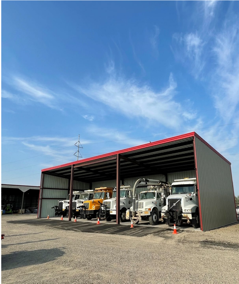
Completed: Public Works Equipment Shed NW 9 th Street
