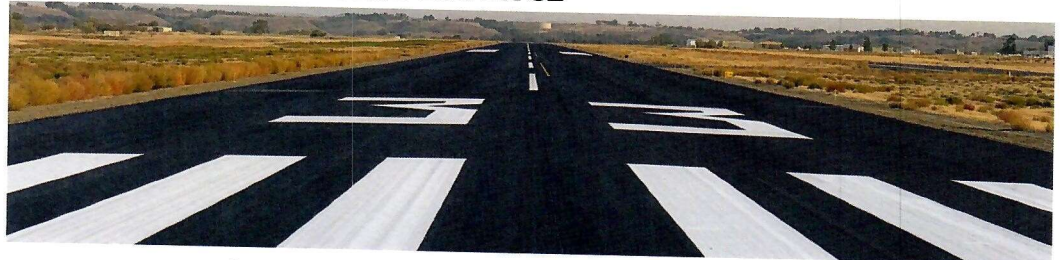
Ontario Municipal Airport | Runway Reconstruction
