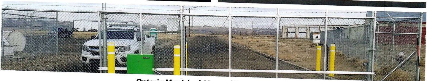
Ontario Municipal Airport | Fence and Gates
