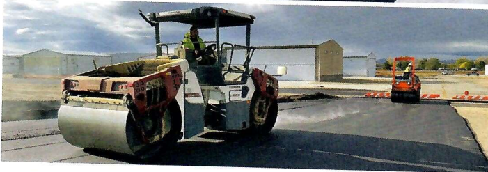
Caldwell Executive Airport | Taxiway Reconstruction
