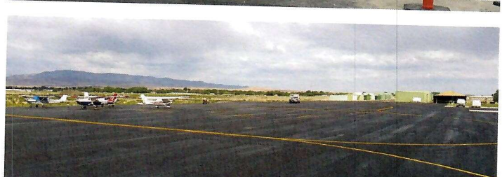
Mountain Home Municipal Airport | Apron Rehabilitation
