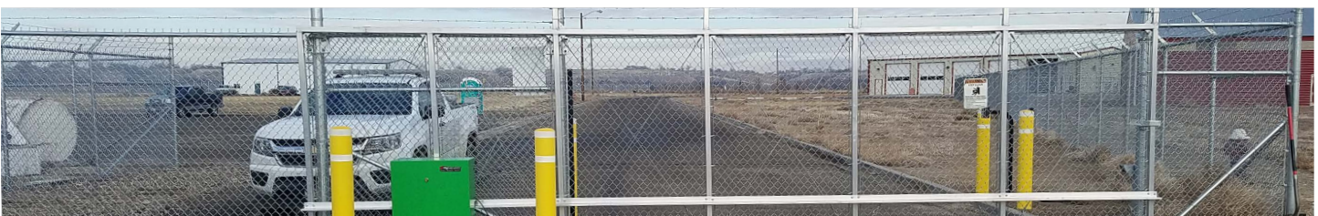
Ontario Municipal Airport | Fence and Gates
