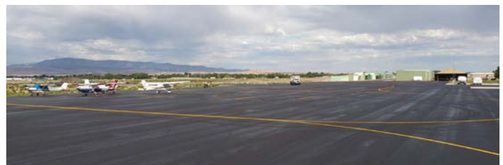
Mountain Home Municipal Airport | Apron Rehabilitation
