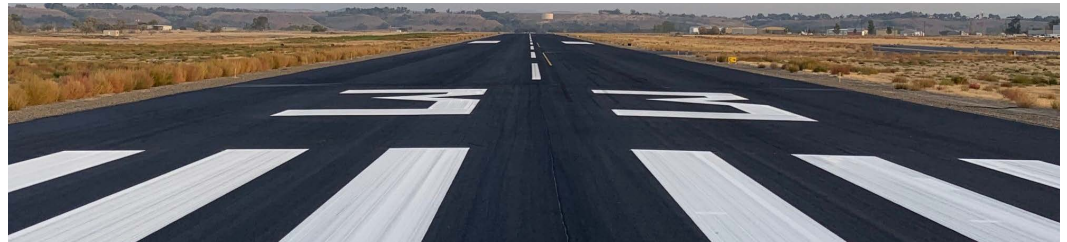
Ontario Municipal Airport | Runway Reconstruction
