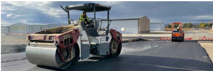
Caldwell Executive Airport | Taxiway Reconstruction
