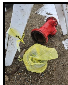
Replacing damaged fire hydrant
