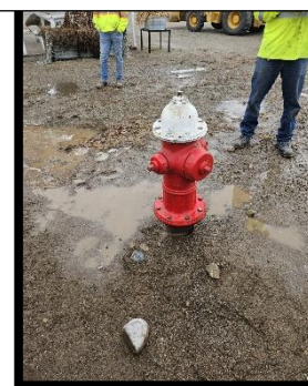
Replacing damaged fire hydrant
