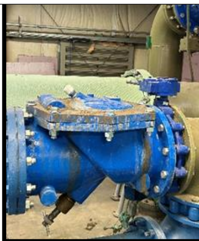
Rebuilt River Pump #2 Swing Check Valve
