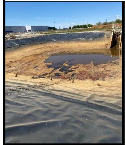
Reinstalled pump in recovery basin 4
