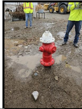
Replacing damaged fire hydrant
