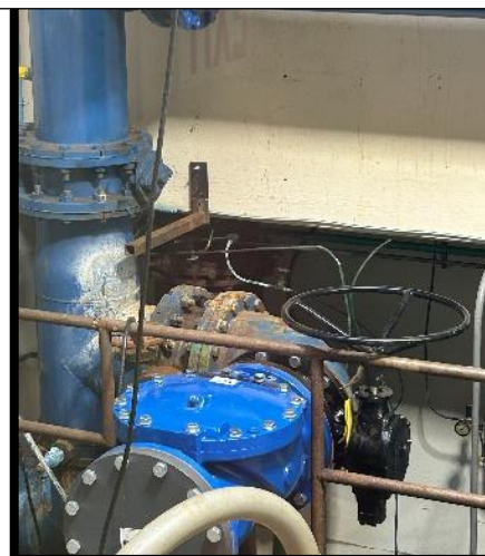
Installed new Butterfly Valve and Check Valve on clear well pump 4 discharge line
