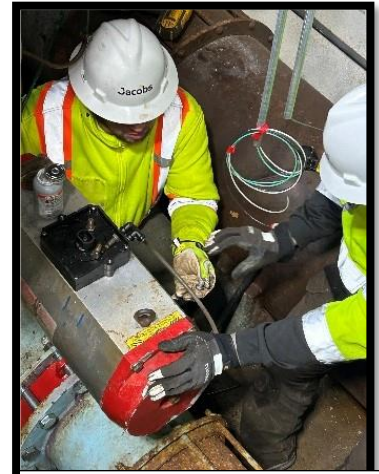
Replaced Filter #1 Effluent Valve
