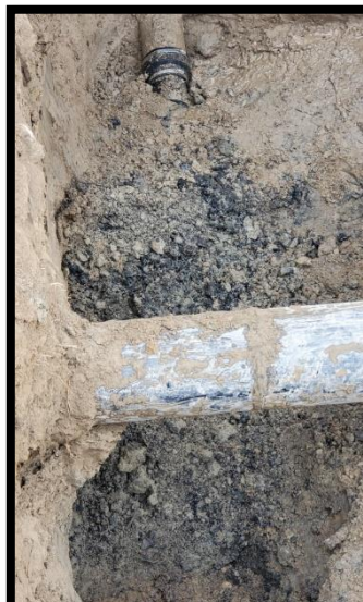
Water and Sewer main exposed for new sewer service to be connected to.
