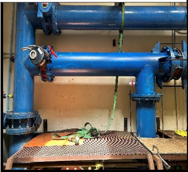
Repair/Replaced backwash piping due to leaks
