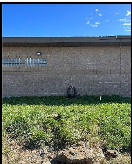
Removal of all identified invasive weeds and dead trees.
