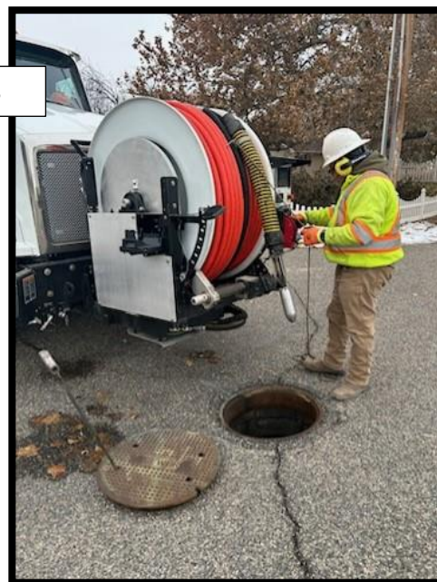
Cleaning sewer lines
