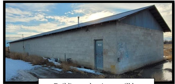
Building at the airport will be demolished for BLM SEAT Base.
