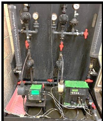
Chemical pump maintenance
