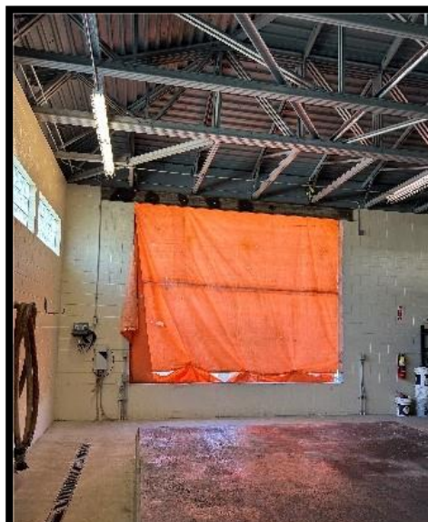
WesTech Expansion Construction Beginning
