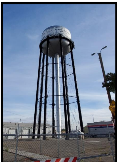
Water Tower meter reading equipment will be installed on.
