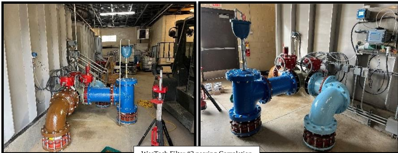
WesTech Filter #3 nearing Completion
