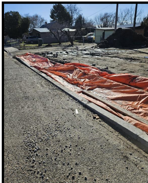
Driveway and sidewalk forms for new residential house.
