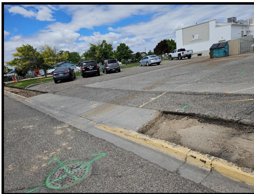
SE 5 th Sidewalk Project
