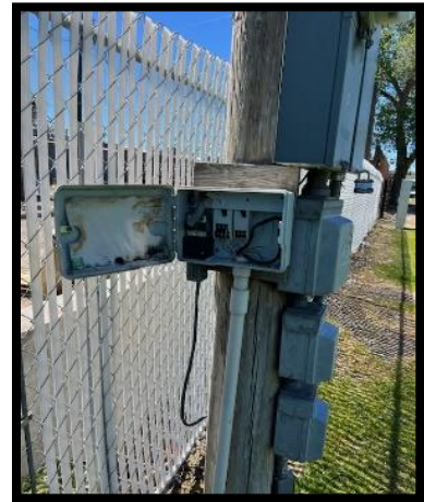
Damaged Water Timer
