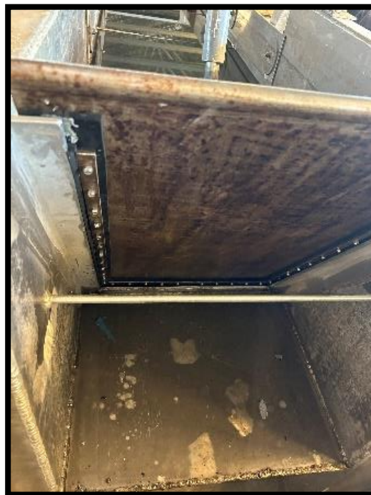
WesTech #3 Waste Gate repaired: Construction Complete
