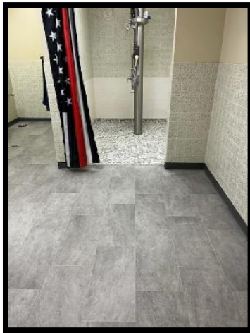
Completed floor in the Fire station restroom.
