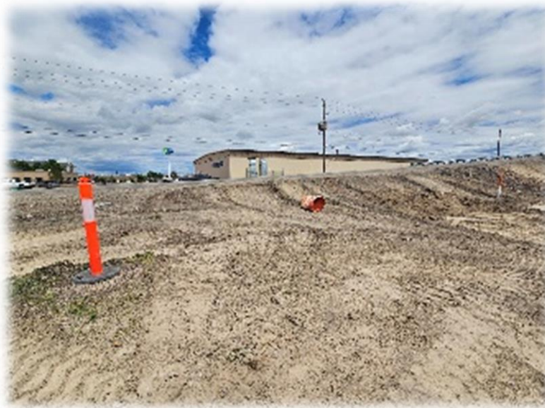
SE 5 th Ave. Sidewalk Project
