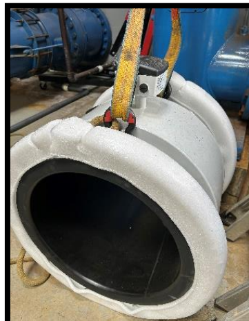
Eastside Flowmeter Replacement.
