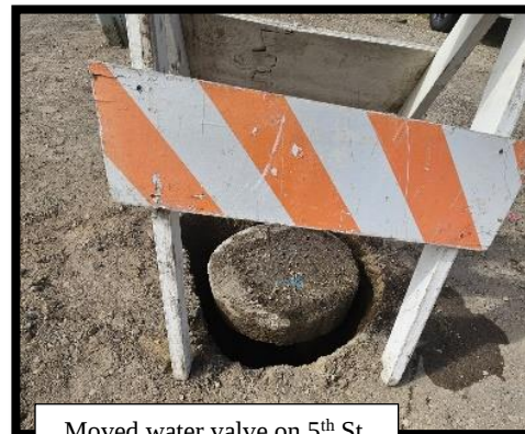
Moved water valve on 5 th St. Sidewalk project.
