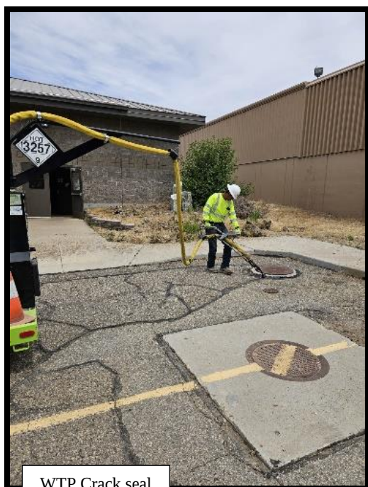
WTP Crack seal
