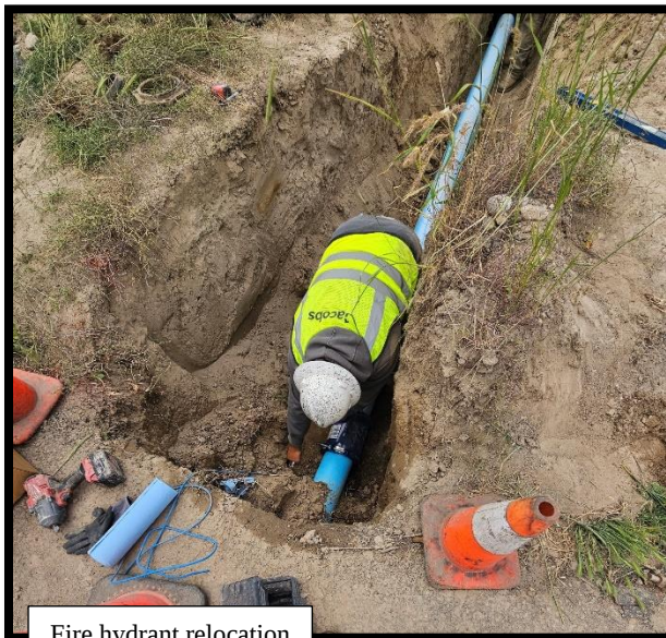
Fire hydrant relocation
