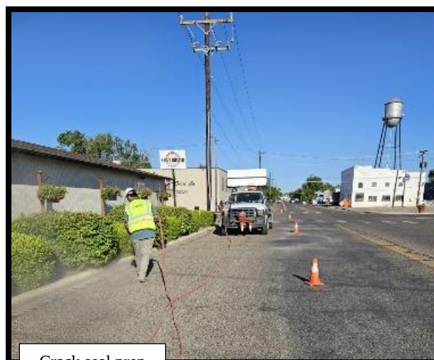
Crack seal prep
