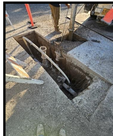
Valve replacement on Pennington Drive.
