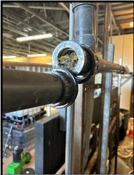
Cleared Microchlor blockage and repaired fill line.
