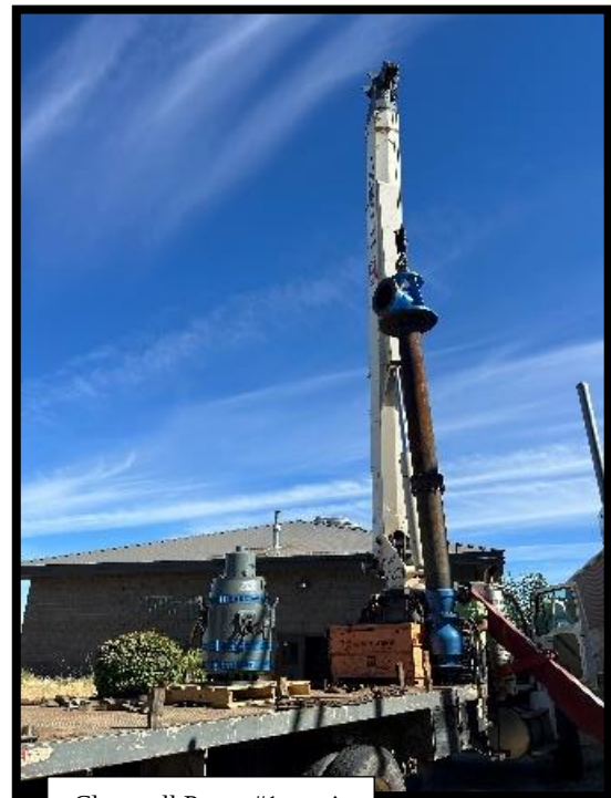
Clearwell Pump #1 repair
