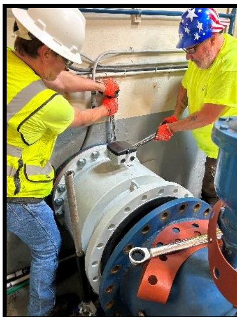
Eastside Flowmeter Replacement
