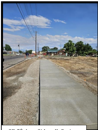
SE 5 th Ave. Sidewalk Project.
