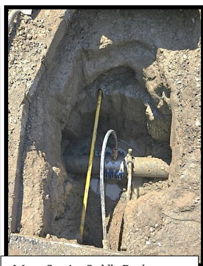
Water Service Saddle Replacement
