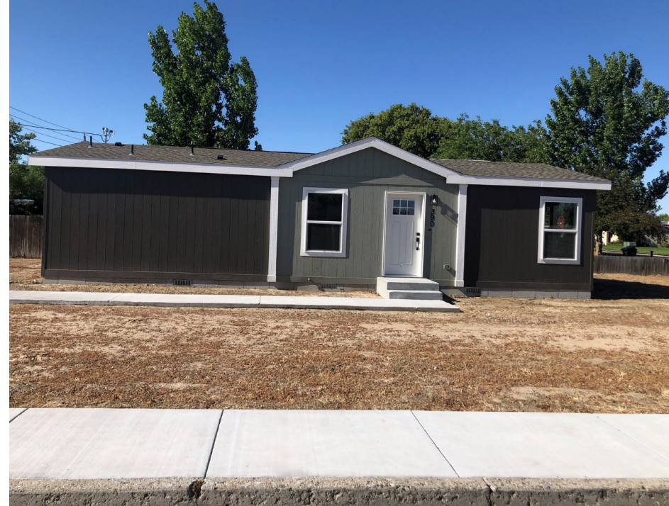
COMPLETED: 390 SW 10 th Avenue
