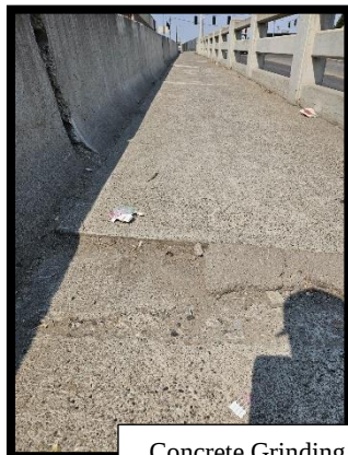
Concrete Grinding on overpass walkway
