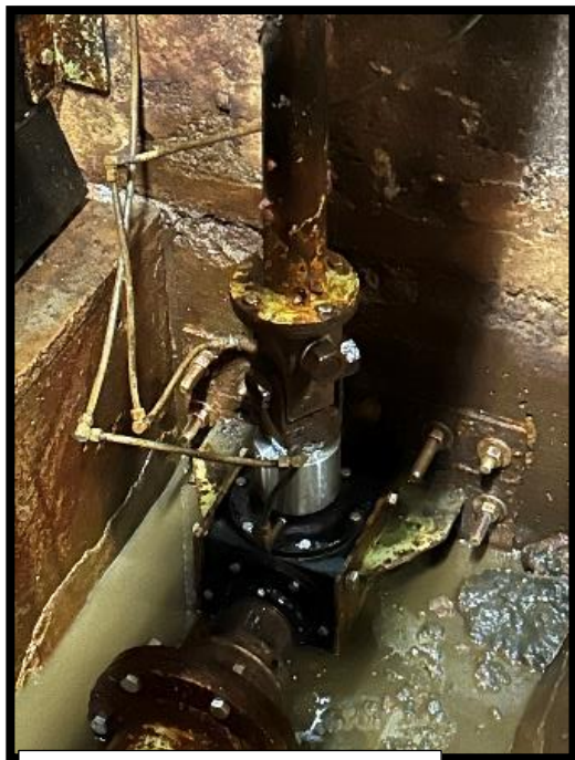
Clarifier #1 Auger gearbox change
