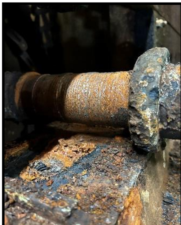
Replaced failed primary drive shaft bearing on flocculator #2
