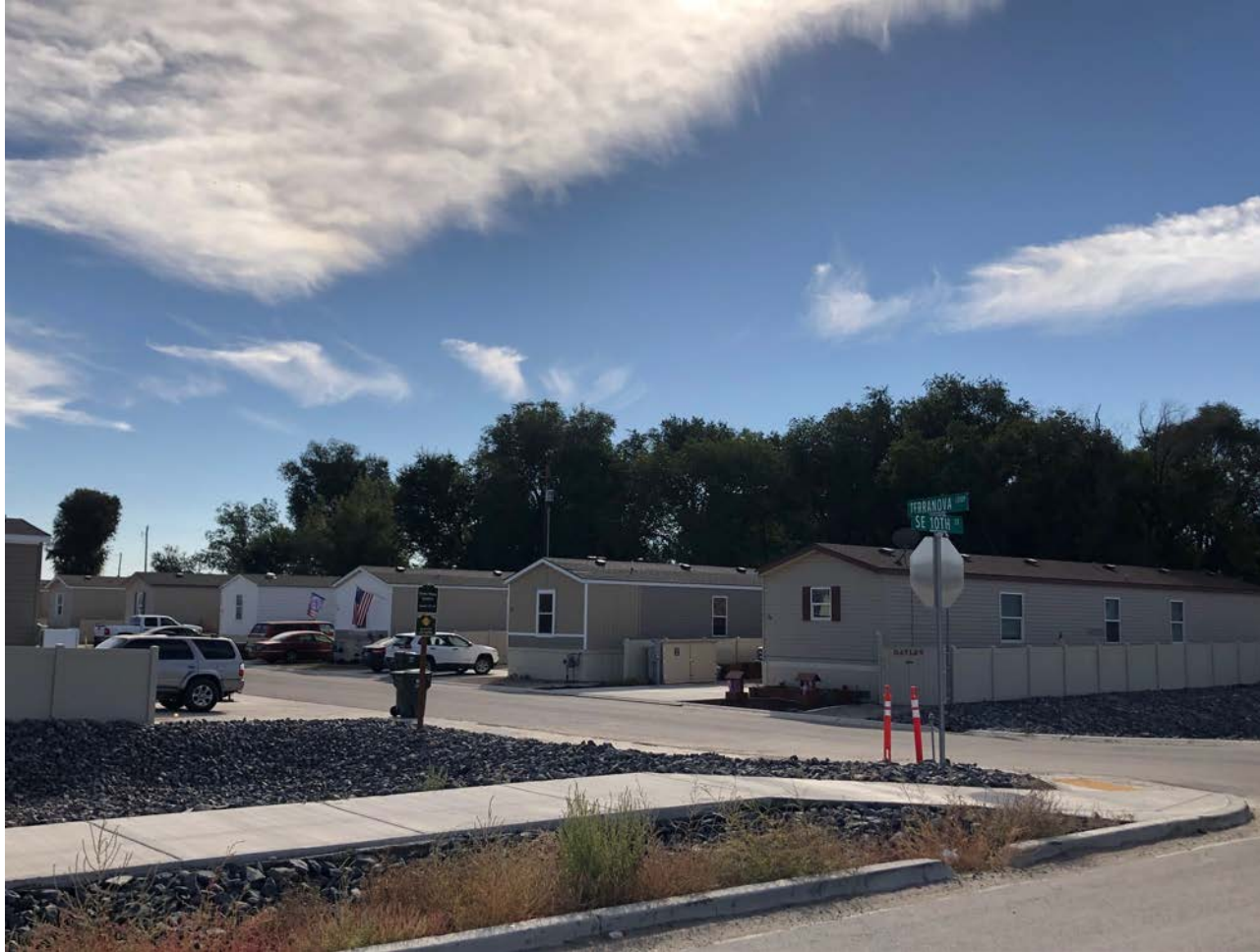
TERRANOVA MOBILE HOME PARK 684 SE 10 th Street 3 more manufactured homes added
