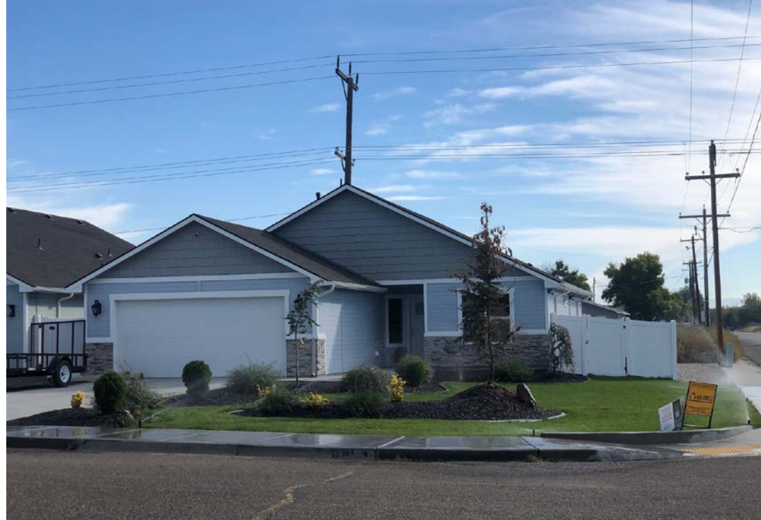
COMPLETED: 798 SE 6 th St
