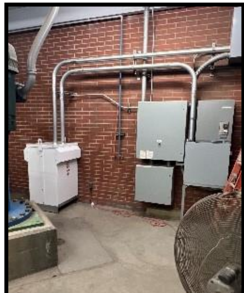
Replaced Harmonic Filter at Eastside Booster Station
