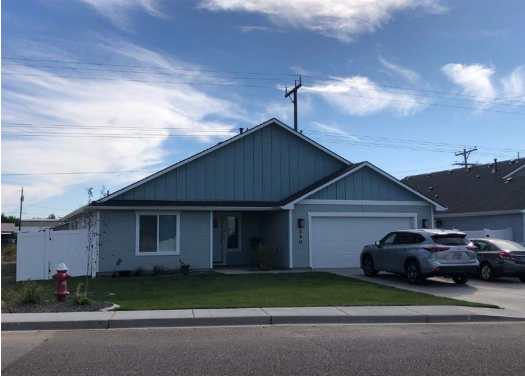
COMPLETED: 790 SE 6 th St
