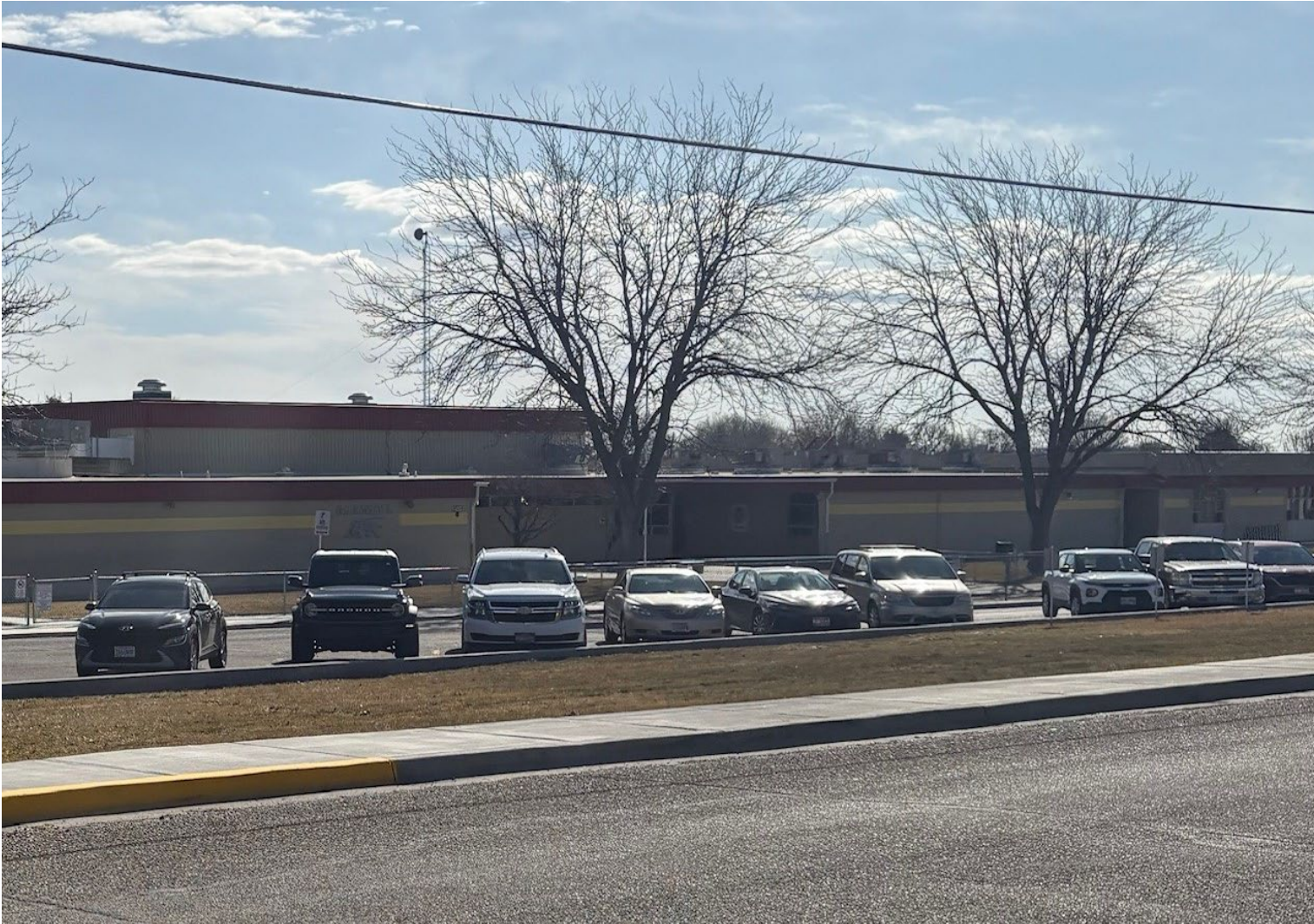
Alameda Elementary School Main Office Interior Remodel
