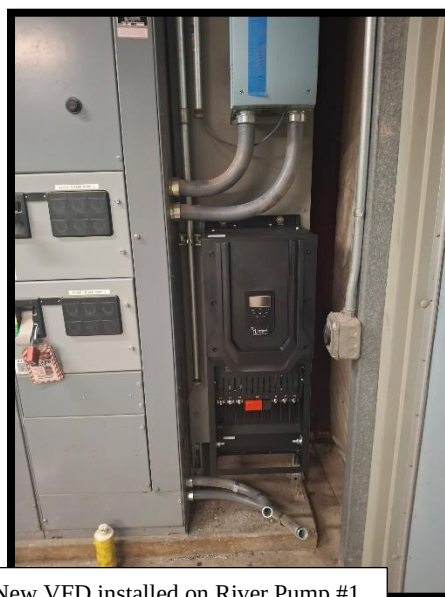
New VFD installed on River Pump #1
