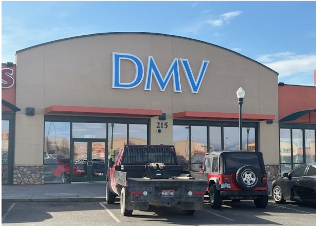
COMPLETED: DMV Office Relocation 215 East Ln N #4
