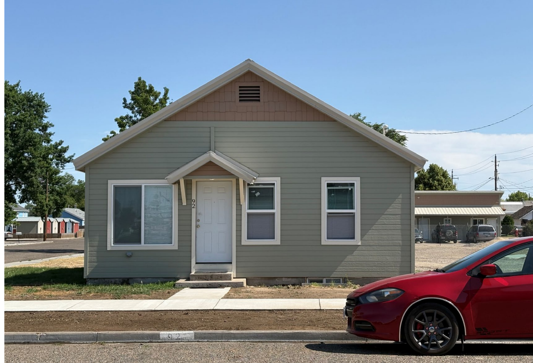
COMPLETED: Remodel of single-family dwelling 92 NW 2 nd Ave
