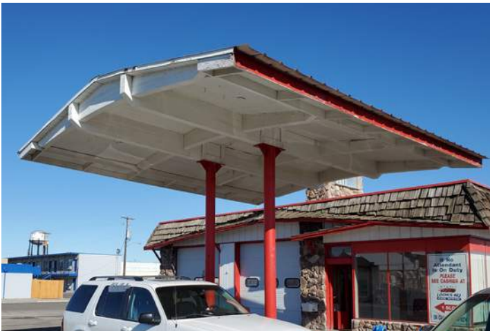
Gas Station Canopy - Period Architecture with Cultural History - Upcycle and Reuse as Shade Structure or Performance Stage
