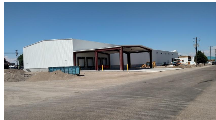
Baker Packing completed
