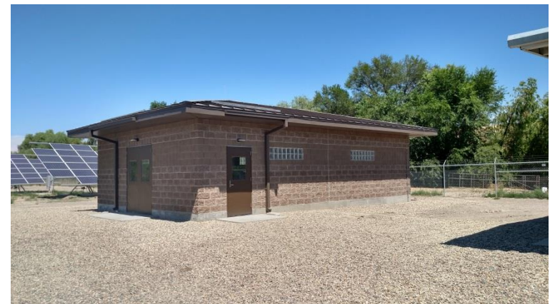
Ontario Water Treatment Plant
