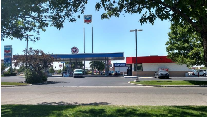
Jackson's Rebuild-Idaho Ave
