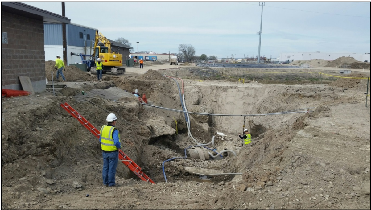
Engineering Division taking GPS points on new pipe for the Chemical Feed Building at the Water Treatment Plant. The new points and lines will be added to the GIS map of underground utilities for the City of Ontario.
