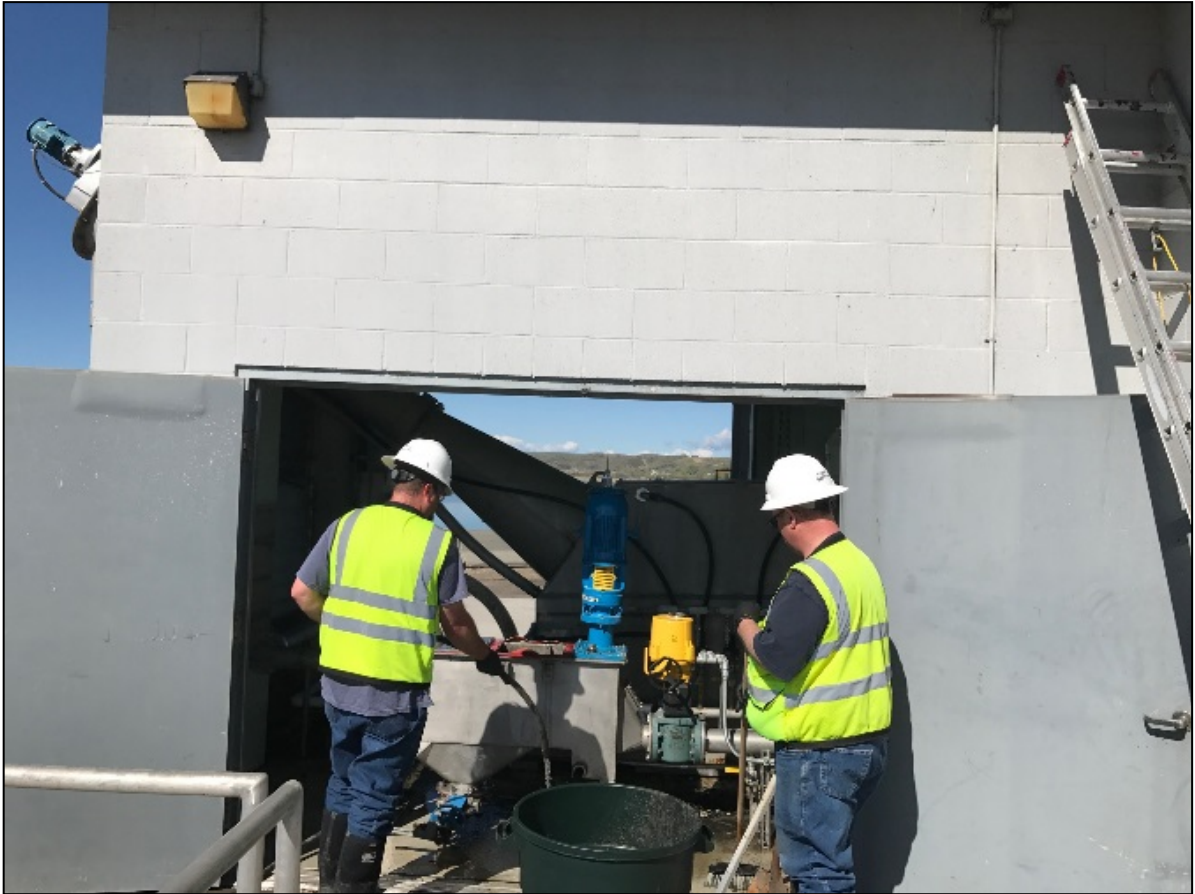
Wastewater Treatment crew cleaning septage receiving station.
