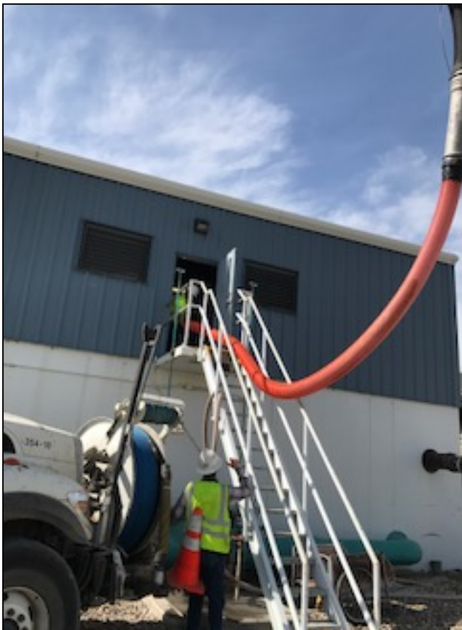
Vacuum hose to remove sand at Water Treatment Plant.
