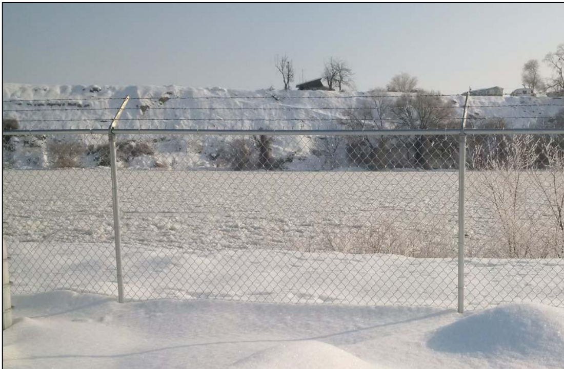
Ice on the Snake River behind the Water Treatment Plant.
