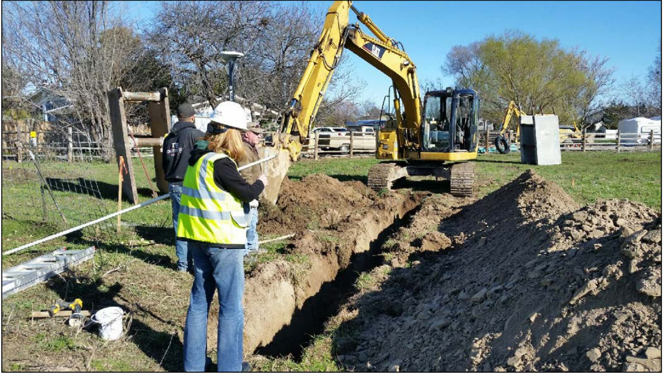
Engineering Technician collects GPS coordinates at a new sewer and water connection for a new residence.
