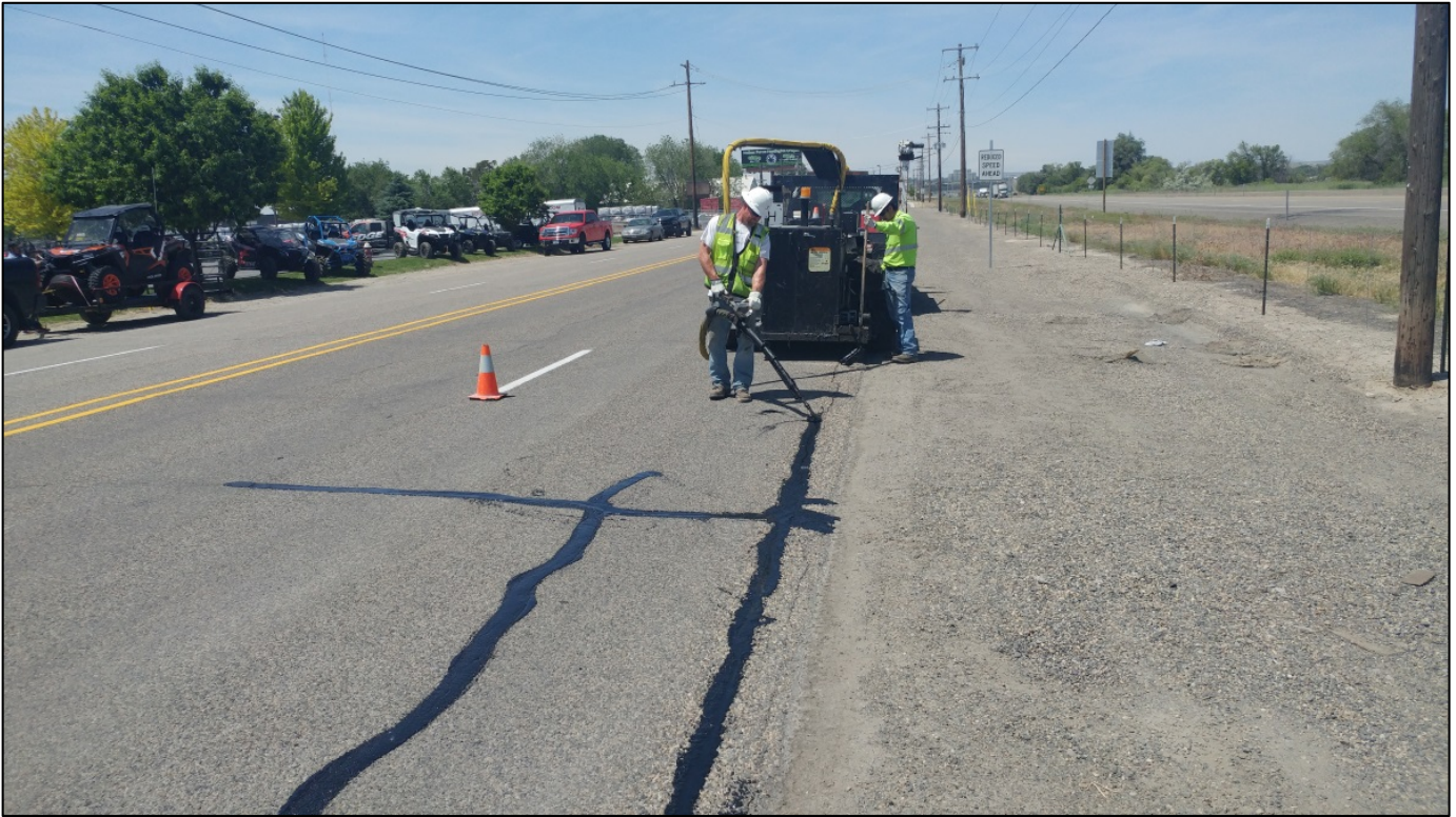
Above, Field Services Crew crack sealing along North Oregon Street in preparation for the summer's chip seal project.
