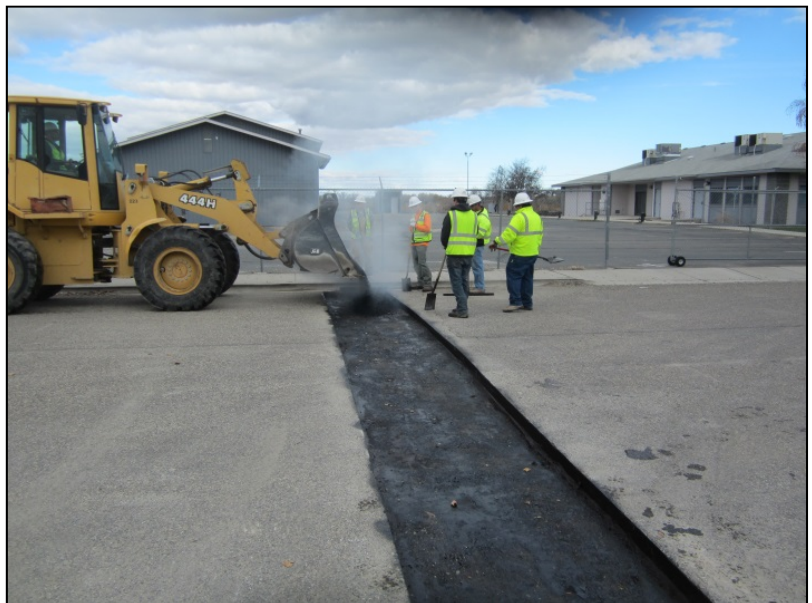
Field Services Crew patching back asphalt – a total of 21 tons around Ontario – before the plant shut down for the winter.
