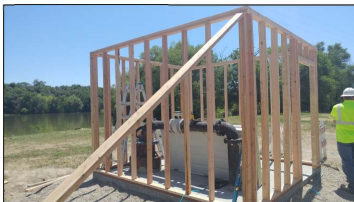
Building the walls for new well house Well No. 17.
