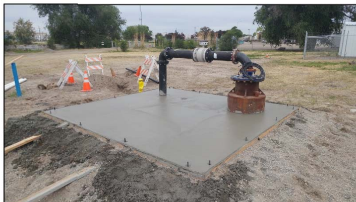
Finished concrete pad for Well No. 17.
