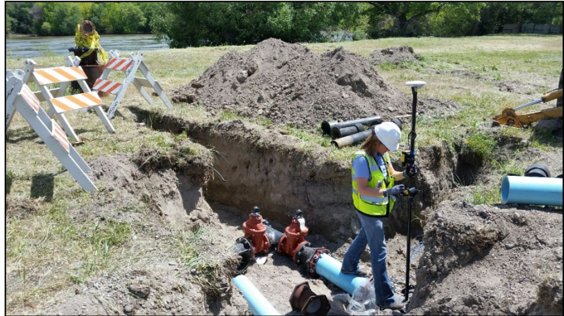
Engineering Technician collects GPS coordinates on newly installed valves at the Water Treatment Plant for Well No. 17.
