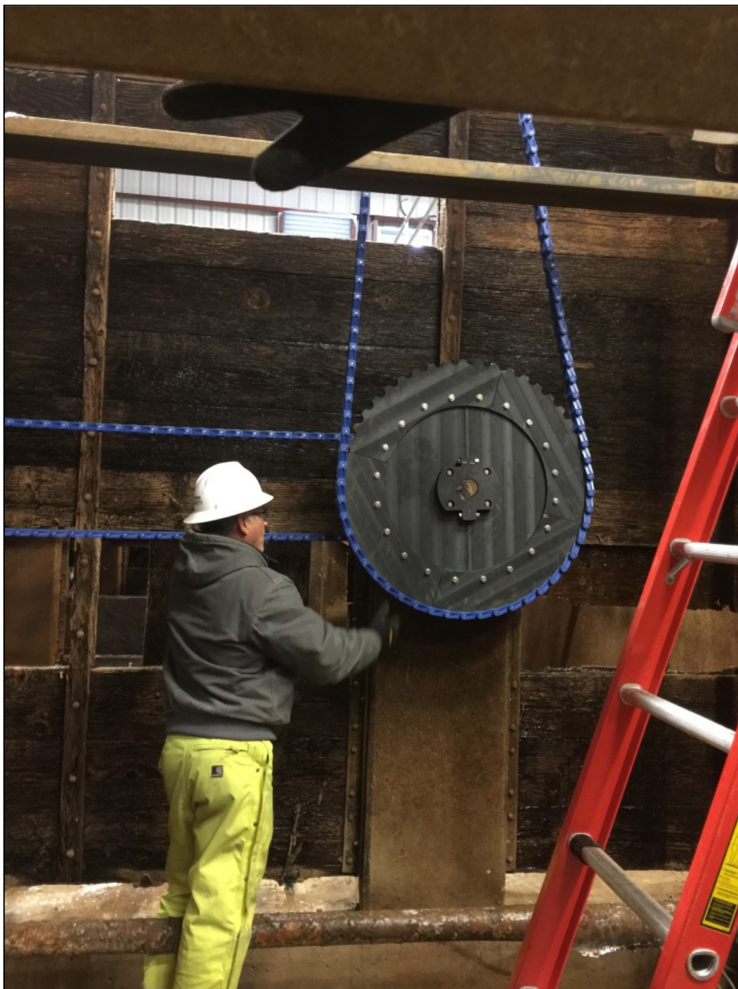
Water Treatment Plant Operator repairs a chain.
