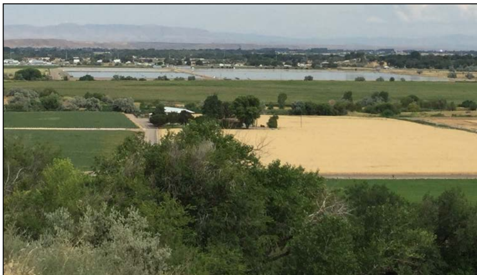
View of the Wastewater Treatment Plant lagoons from the Bench Reservoir.
