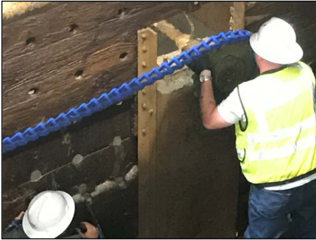
Water Treatment Plant Operators replacing the drive chain for clarifier No. 2 flocculator.
