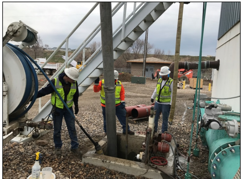
Field Services Crew Seth Blackburn, Raymundo Rodriguez and Operator Robert Crites clearing the drain line of clarifier No. 1 "old plant".
