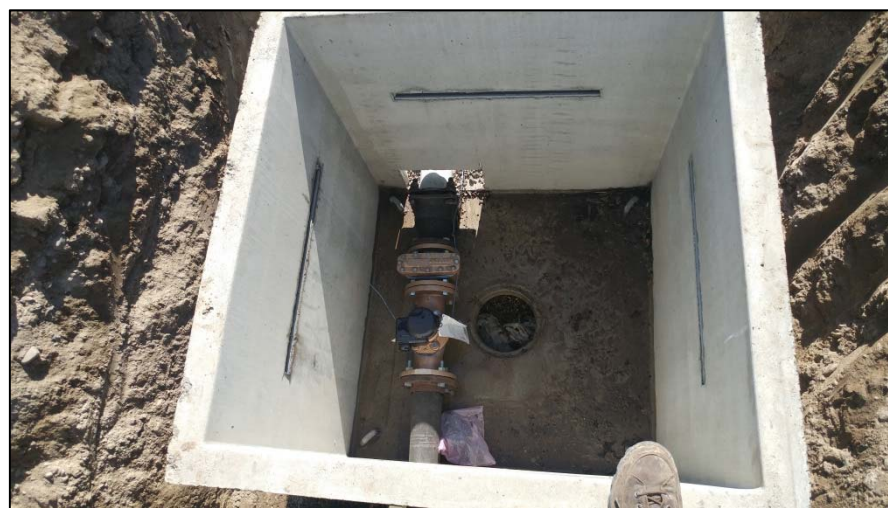
Water meter installation completed for the BLM.
