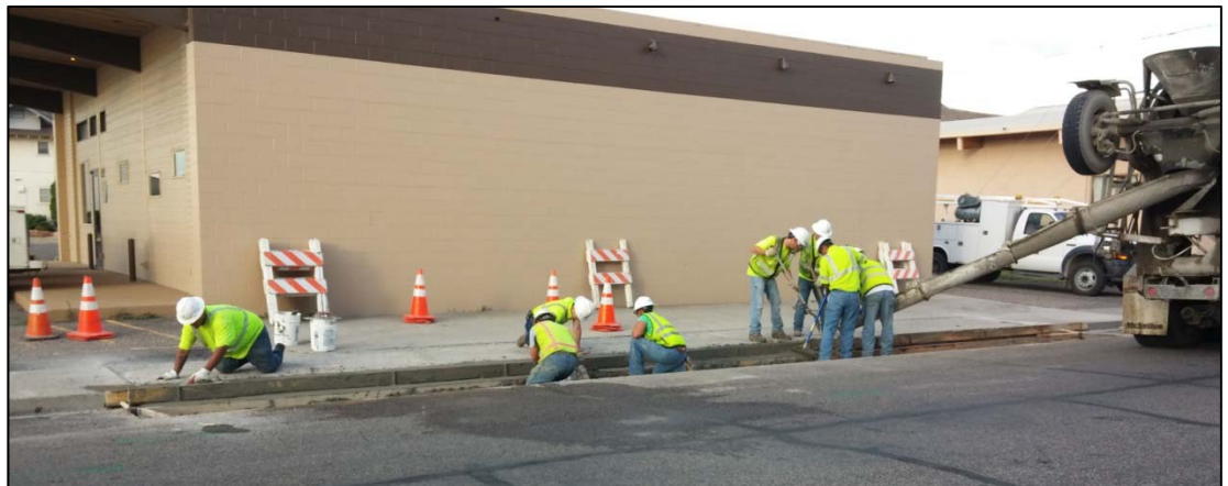
Field Services crew pouring concrete curb and gutter on NW 2 nd Avenue.
