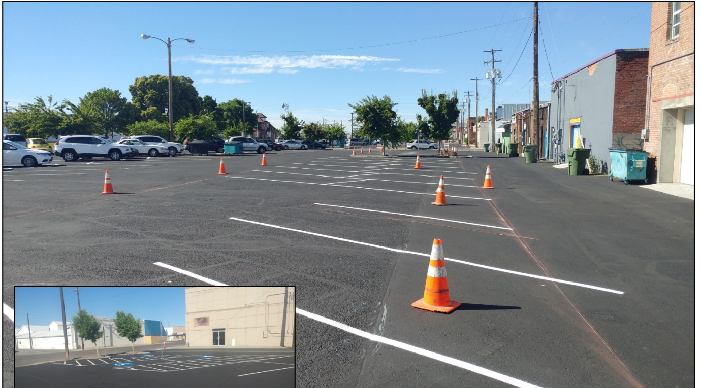
Field Services Crew managed the slurry seal of the City parking lots downtown and restriped the parking spaces.
