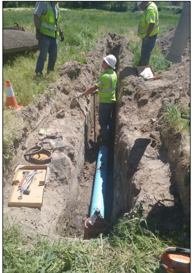
At right, Field Services Crew installing new water valves to new Well No. 17 at the Water Treatment Plant.
