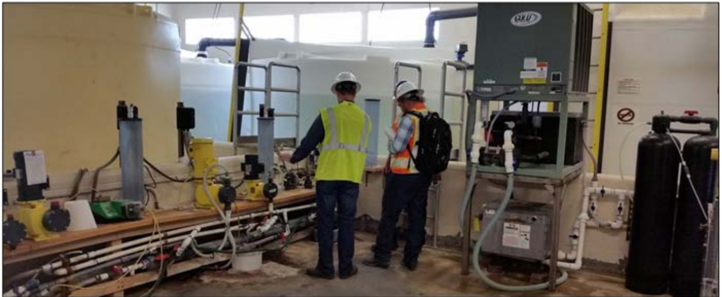
Water Treatment Plant Crew held a preconstruction meeting for the 2016 Chemical Feed Improvements project.
