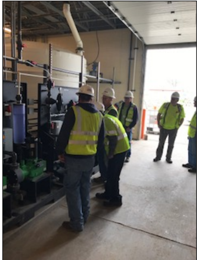
Crew running pump calibration curves for the new ferric and poly chemical pumps and chlorine chemical pumps.
