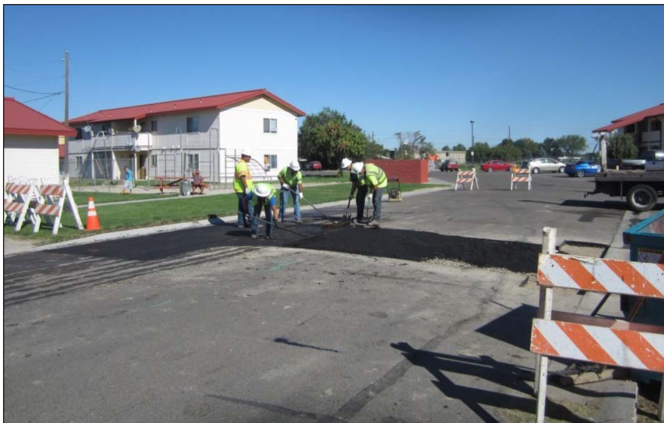
Field Services Crew patching back asphalt at Sierra Vista Apartments.
