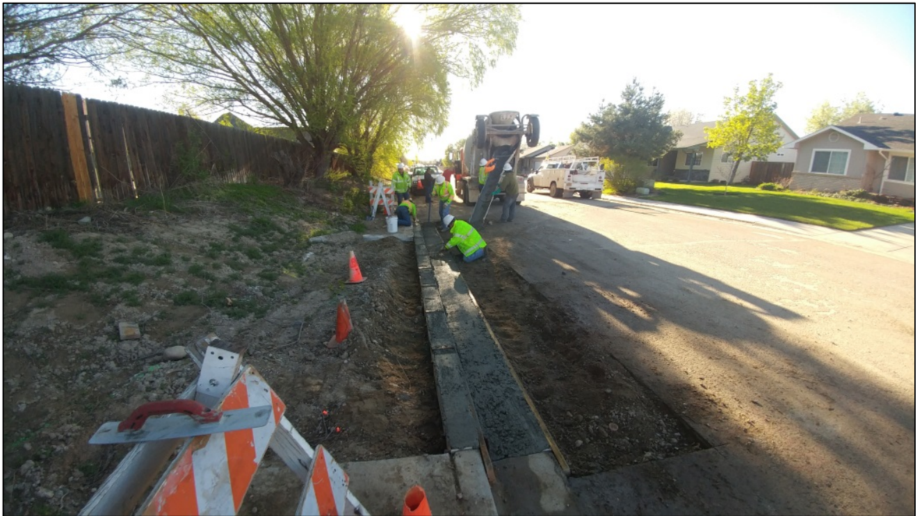
Field Services Crew finishing new concrete curb and gutter along West Idaho Avenue.
