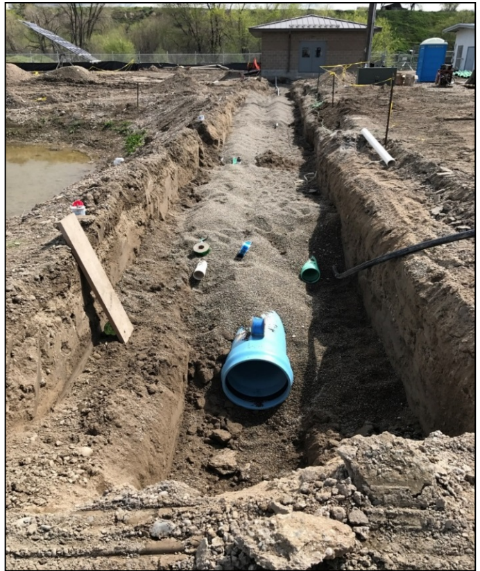
New 20-inch water supply line for the WesTech Treatment Plant.
