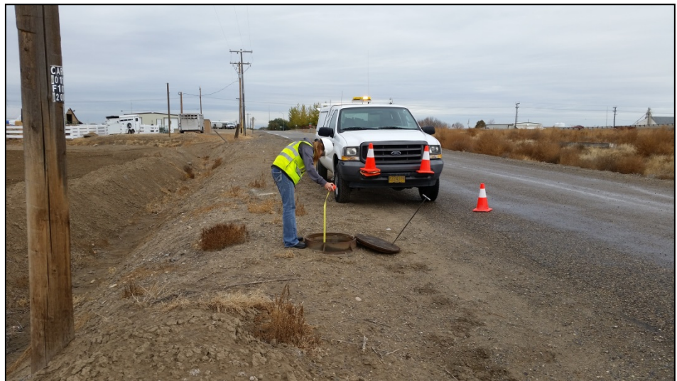
Engineering Technician uses a tape measure to dip a manhole and determine its depth along SW 4th Street, south of SW 18 th Avenue.
