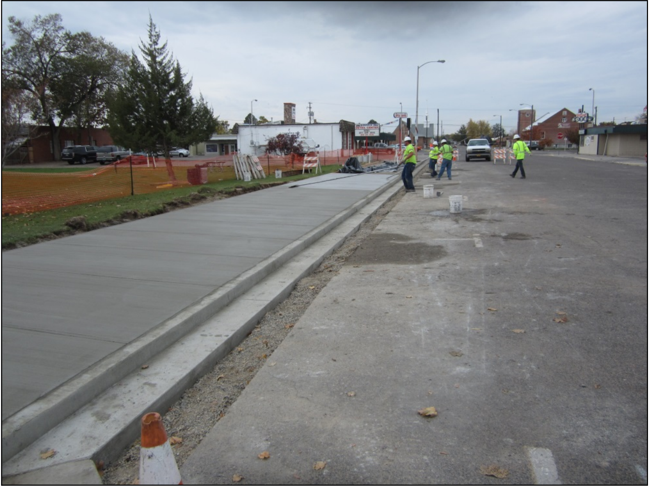
Field Services Crew finishing freshly poured concrete along Moore Park at SW 1 st Street and South Oregon Street.
