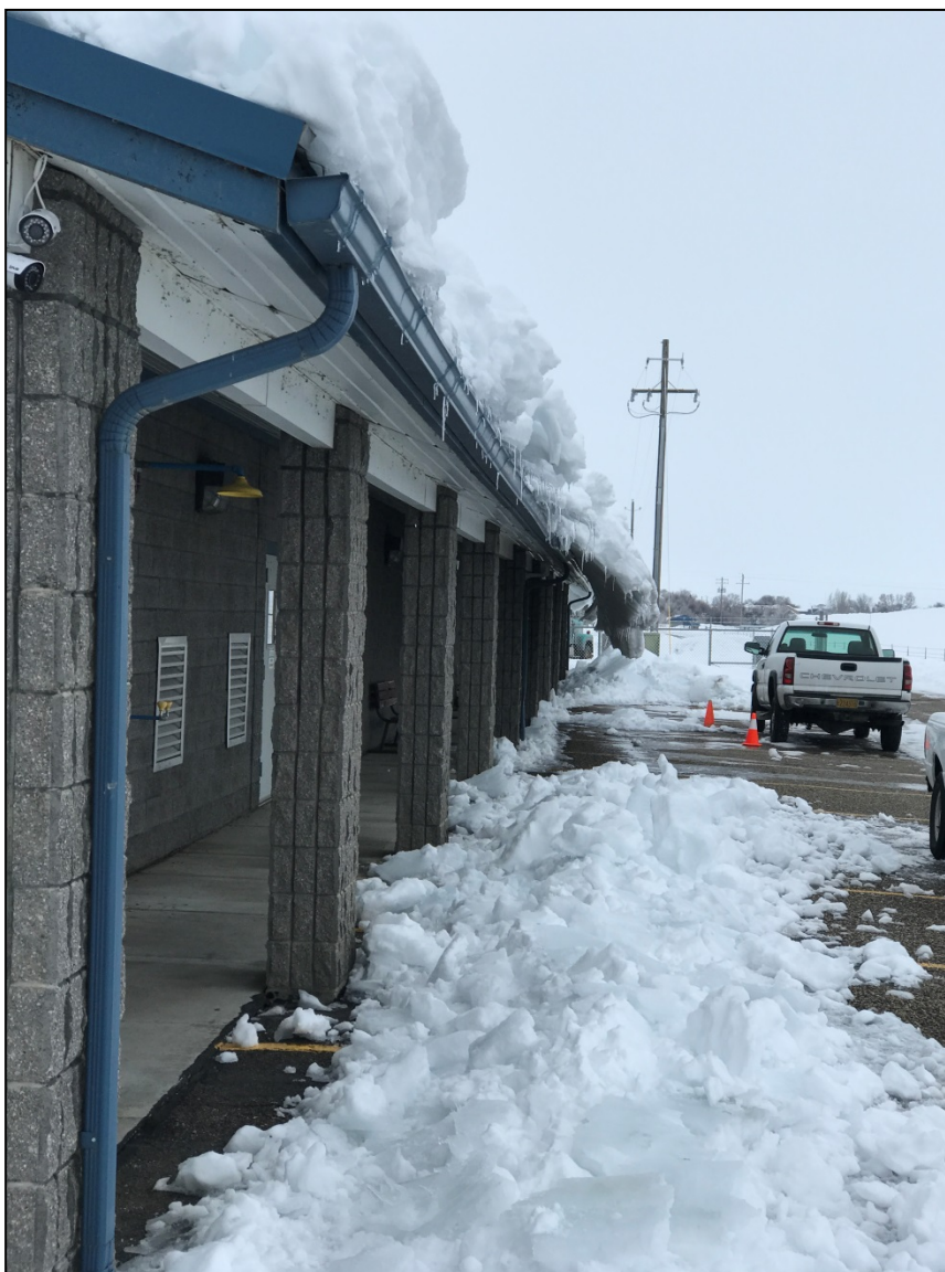
Wastewater Treatment Plant roof snow removal.
