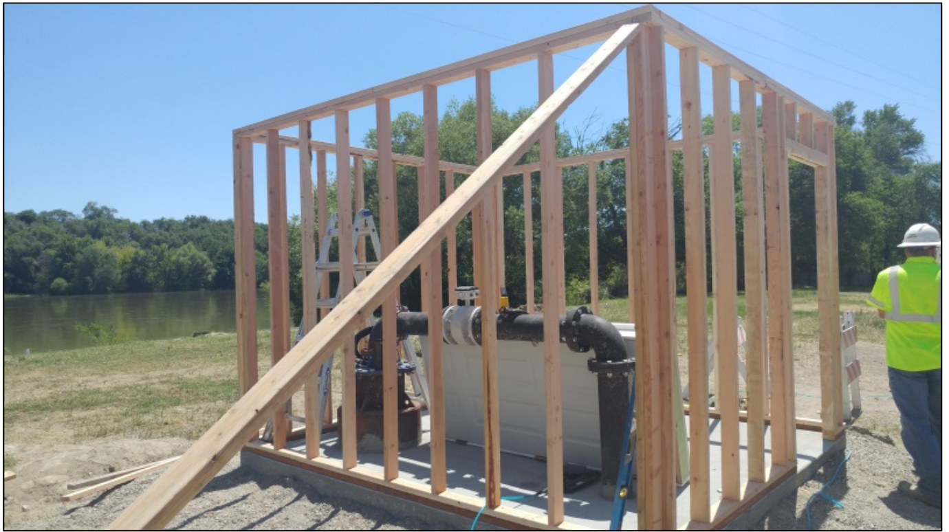
Building the walls for new well house Well No. 17 at the Water Treatment Plant.
