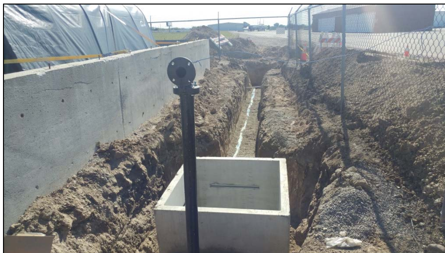
Water meter installation for the Bureau of Land Management at the Ontario Municipal Airport.
