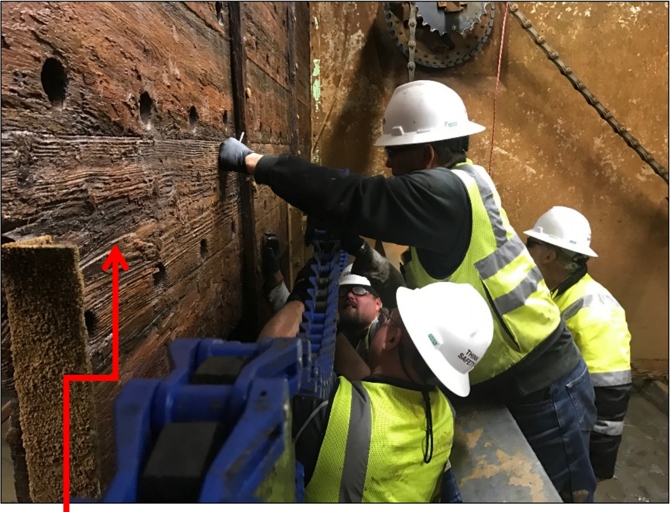
Water Treatment Plant crew repairing chain and sprockets in clarifier No. 2. Redwood bafflewall to be replaced later this year.
