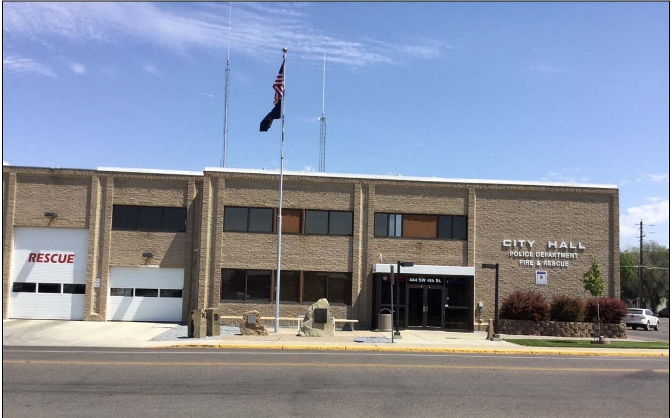
Ontario City Hall – Police Department plus Fire and Rescue.
