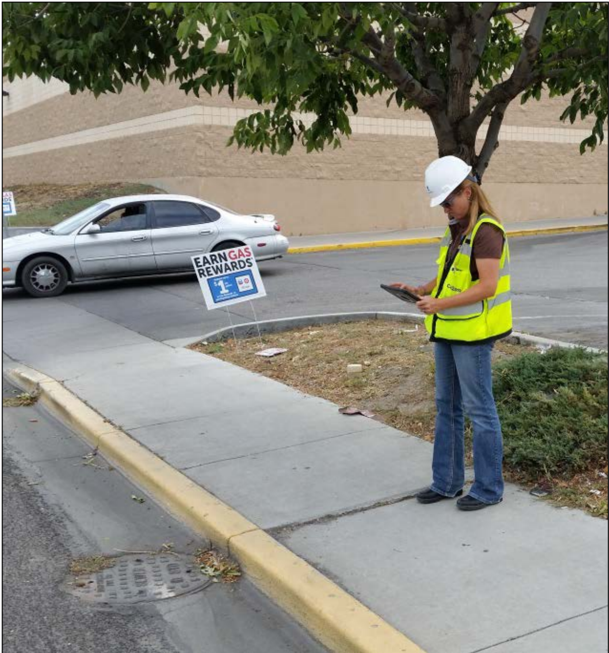
CH2M Engineering Technician inspects sidewalk at Albertson's in Ontario following a trip and fall complaint.
