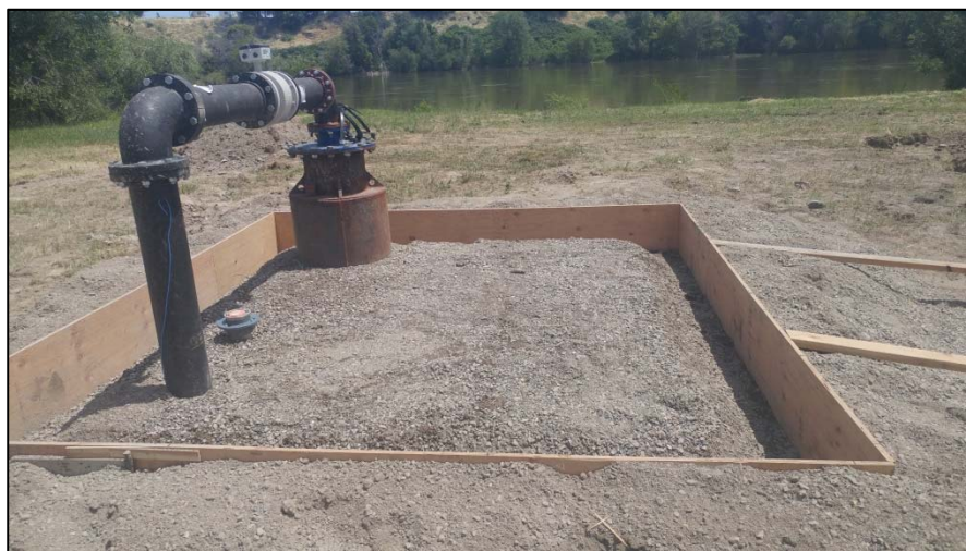
Field Services Crew forms the foundation for new Well No. 17.
