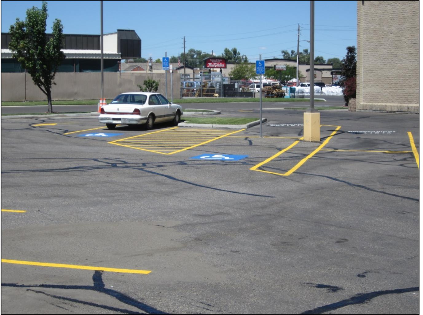
Field Services crew crack sealed and repainted parking stripes at City Hall (top photo) and Optimist Park on North Verde Drive (bottom photo).
