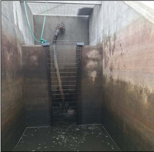
Recovery pond cleaning by Water Treatment Plant operators.
