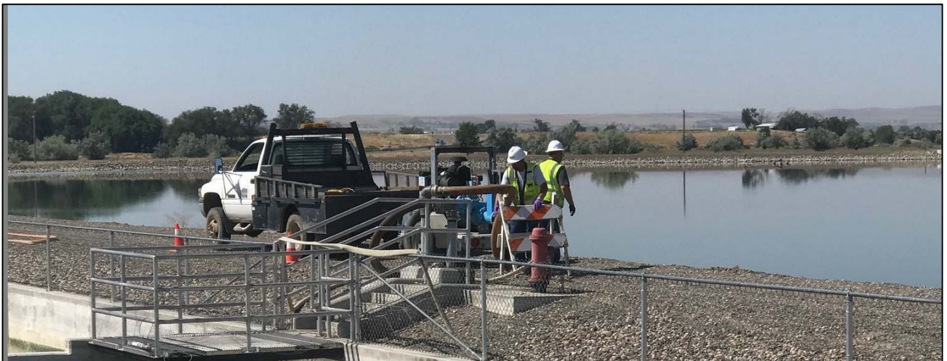
Chlorine contact basin No. 2.
