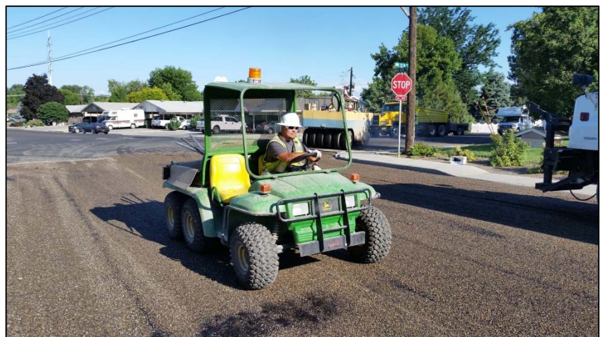
Field Services Crew chip sealing NW 2 nd Avenue and NW 4 th Avenue.
