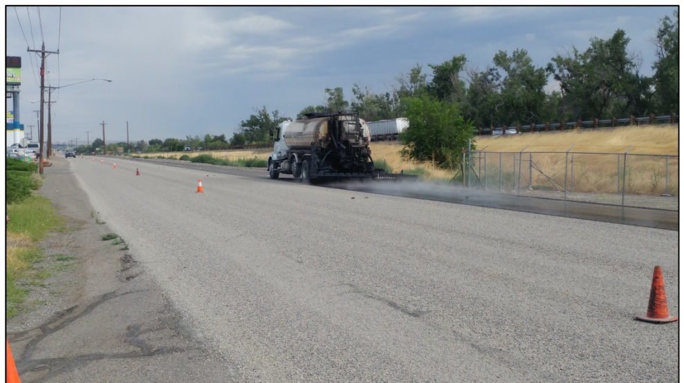
Field Services Crew chip sealing North Oregon Street.
