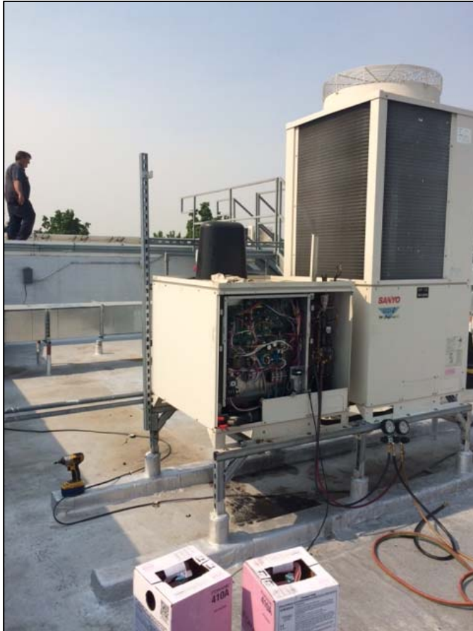
Hobson working on the HVAC system at Ontario City Hall.
