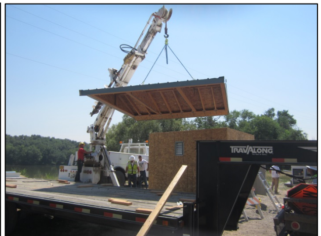
Water Treatment Plant Well No. 17 new well house construction.
