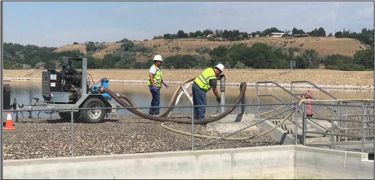
Cleaning chlorine contact basin No. 1 at WWTP.
