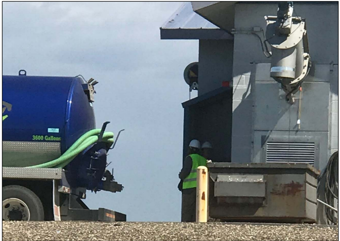
Septage Receiving Plant receiving a load.
