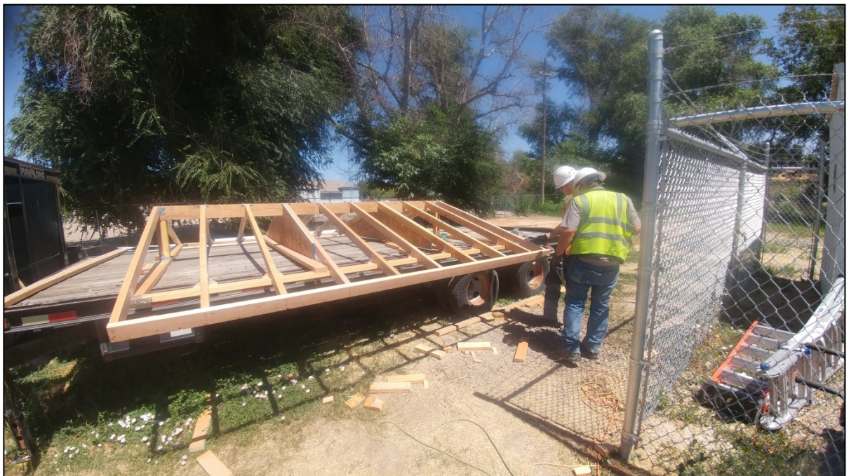
Water Treatment Plant Well No. 17 new well house wall construction.
