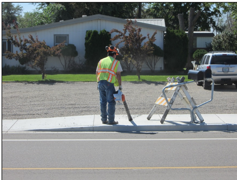
Field Services crew blowing chips off sidewalks.
