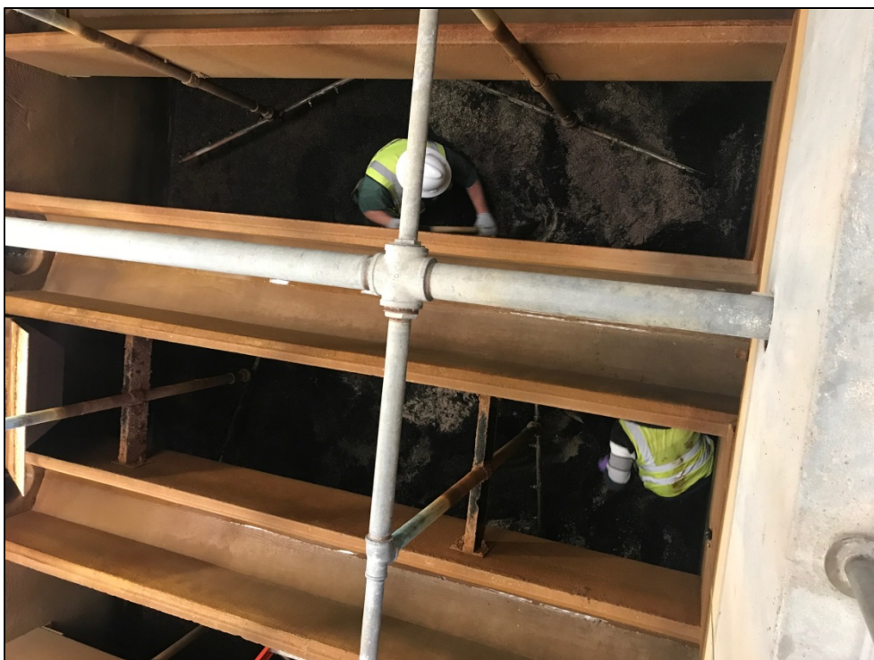
Water Treatment Plant employees making repairs to filter No. 2 at the Water Treatment Plant.
