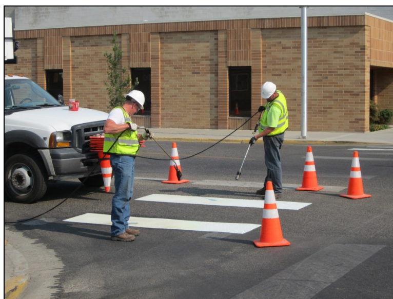
Field Services crew hot taping crosswalk bars.
