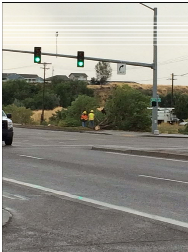
Contractors taking out street trees along East Idaho Avenue in front of Dutch Brothers and Big 5.
